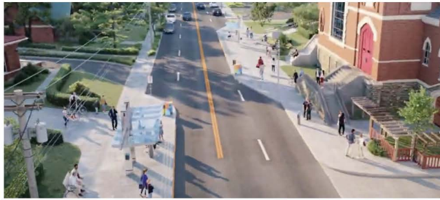
Example of permanent narrowing of traffic lanes.
