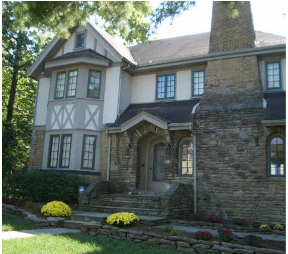
The front of the building has remained relatively unchanged. Where all the construction is still happening is in the back where students will be entering from the elementary woods.
